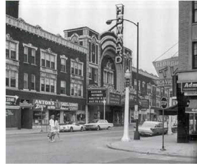
Howard Street Theatre Opened in 1917. By 1975 it was closed and by 1999 the auditorium was razed but the facade and outdoor lobby was saved.
