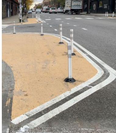
Example of a paint and post bump-out.
