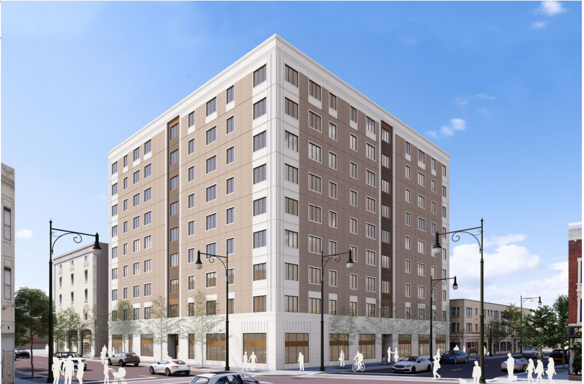
Southwest Corner View
