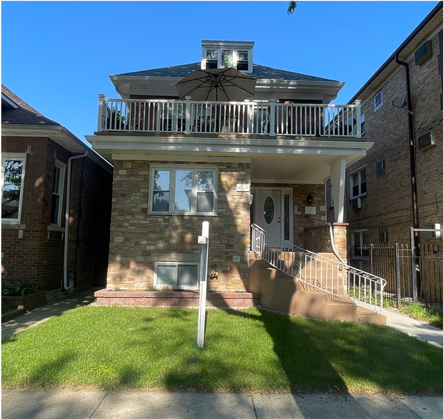
FRONT ELEVATION LOOKING WEST
